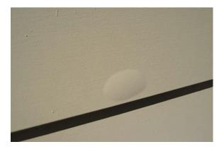
Typical blistering when delamination of older paint coats under new paint coating occurs
